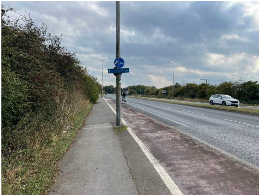
Photo 3: Segregated Foot/Cycleway Along the A1079 Beverley Road
